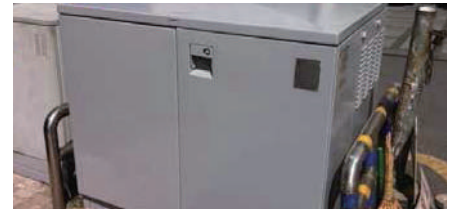
After removing the rust
