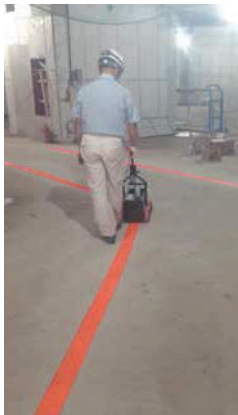
Safety-line work in the construction site
