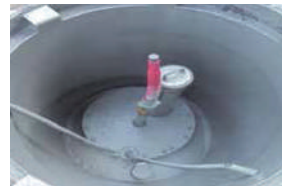
Manhole of the gas station oil tank
