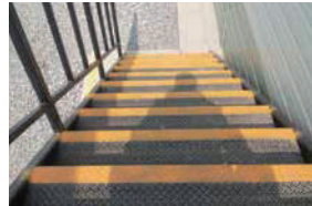
Applying to temporary metal staircase
