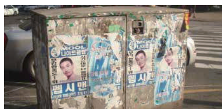
Before applying Anti-Stickers Paint
